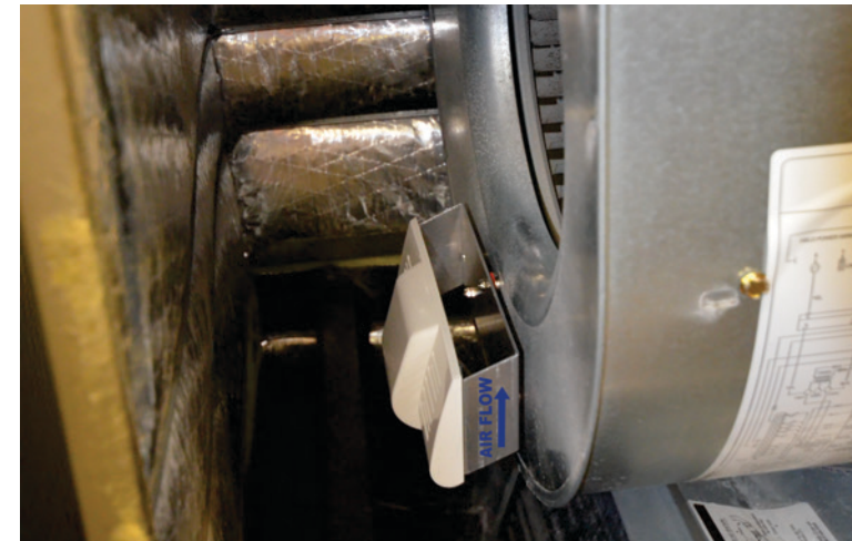
RGFClear Sky™DM mounted to blower housing
